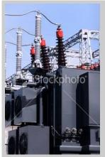
A huge advantage of generating electricity as AC is that it allows us to use transformers, which allow us to step-up or step-down and AC voltage to any desired value.
