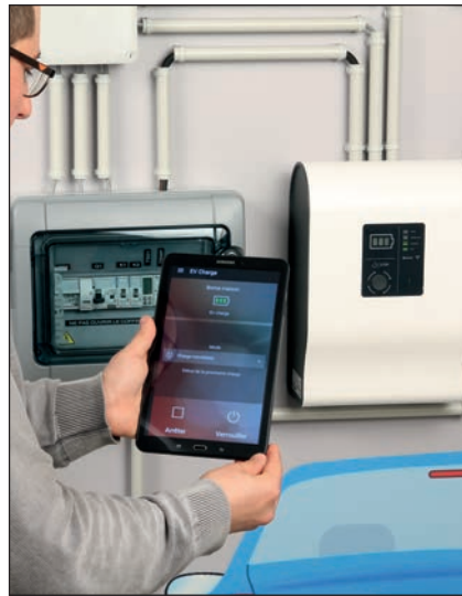
The charging station communicates via Wifi or Bluetooth. The locally created wifi network is specific to the model. It is isolated from the WiFi network of your building.
